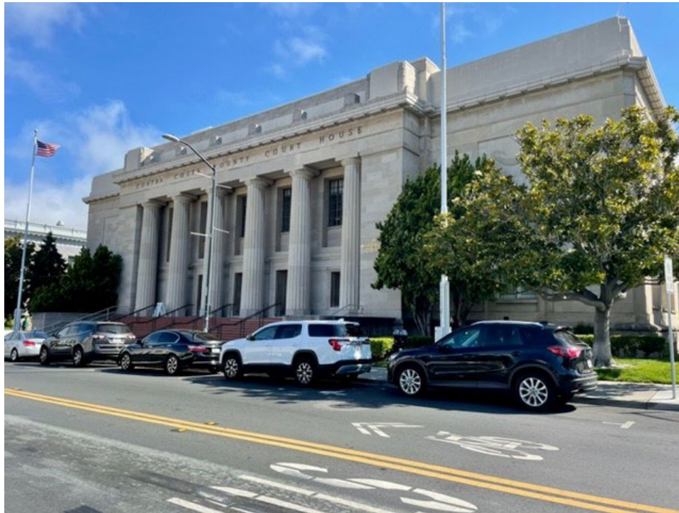
Contra Costa County Courthouse
