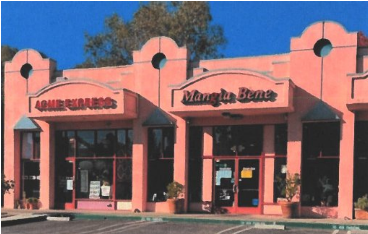
Figure 2 – View of Subject Site From 'X'
