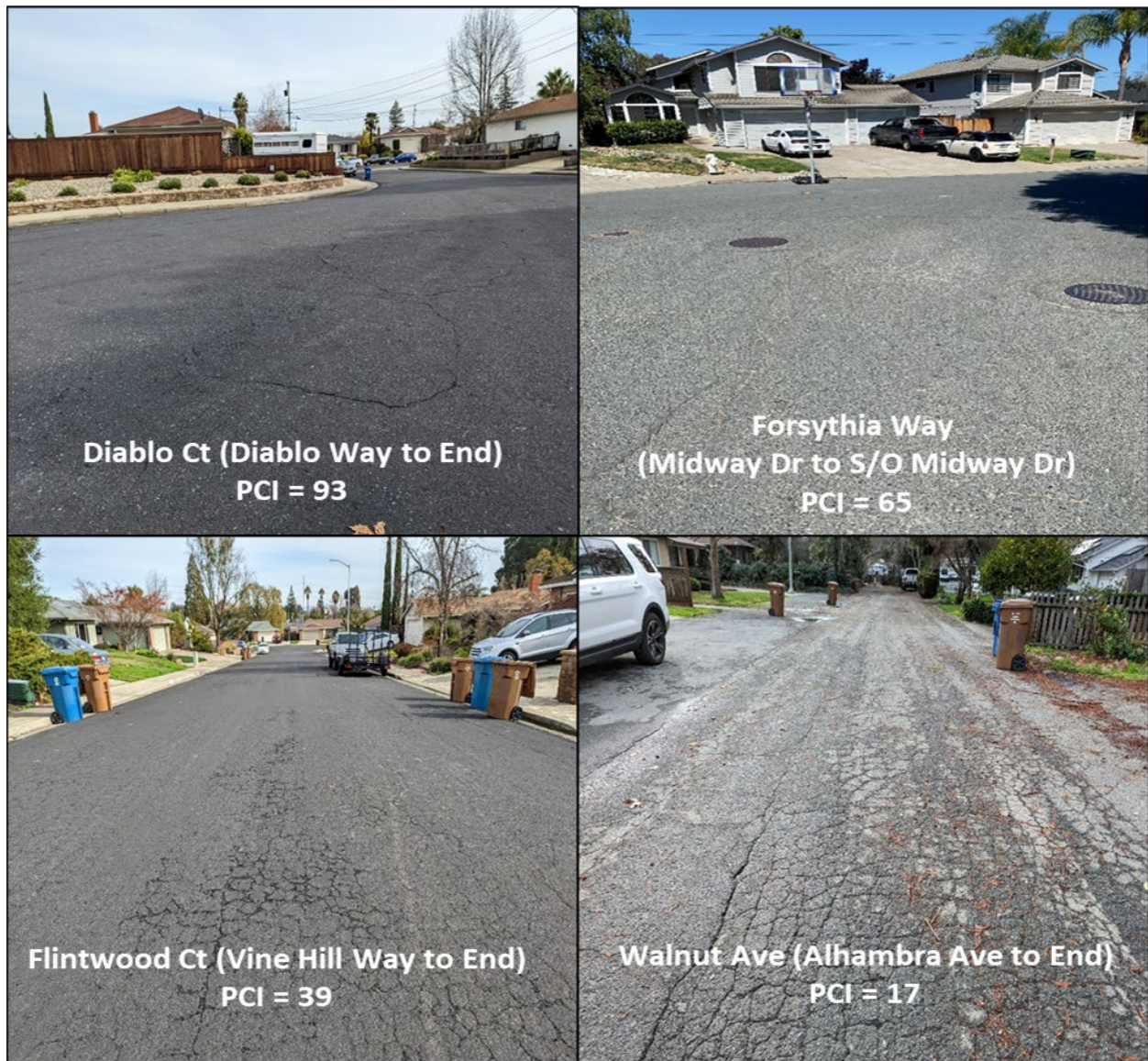
Figure 1. Examples of Streets with Different PCIs
