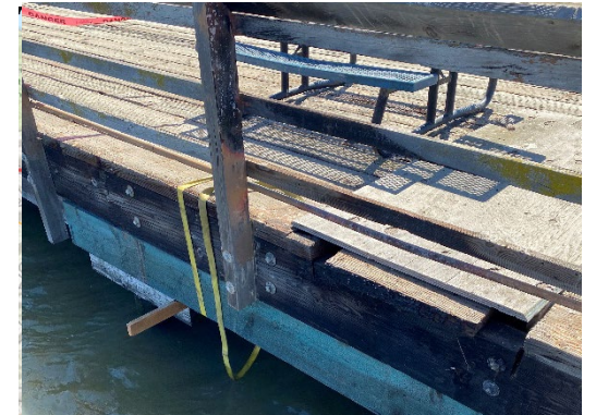
Fishing Pier Repairs
