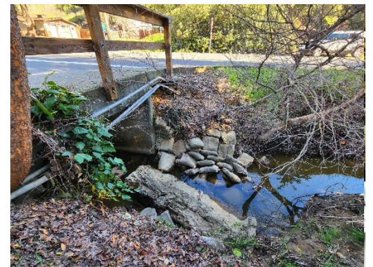
Citywide Bridge Repairs
