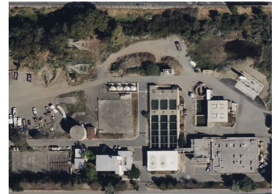
Water Treatment Plant
