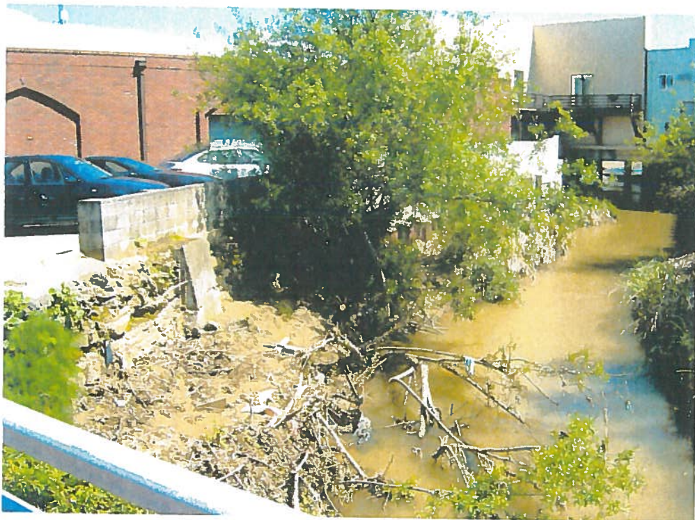
1 to 2 feet of sediment deposited on east bank at Escobar Street from December 30-31, 2005 storm
