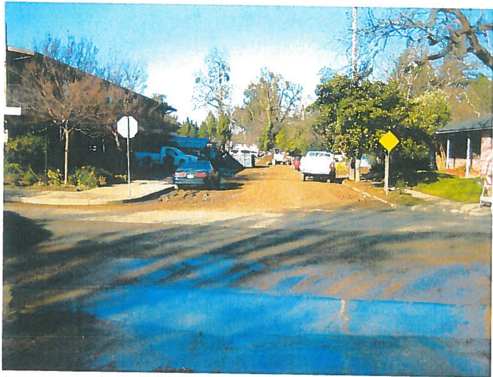
Sediment deposited along D Street and in the curb and gutter on Castro Street
