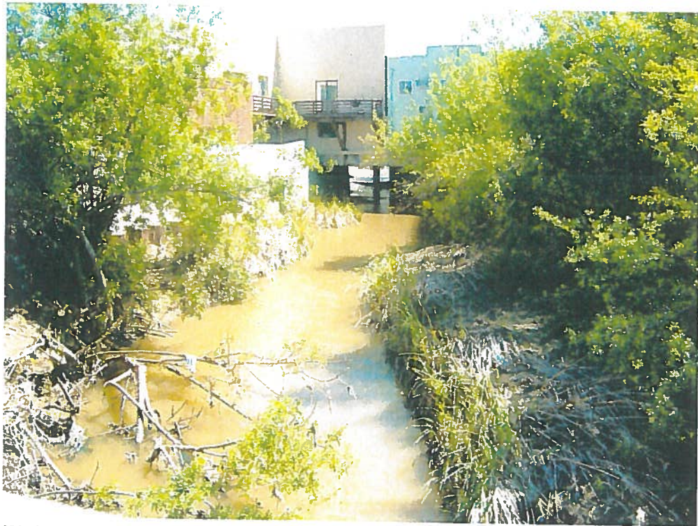
Wetland vegetation bent over and up to 1 foot of sediment deposits on west bank at Escobar Street
