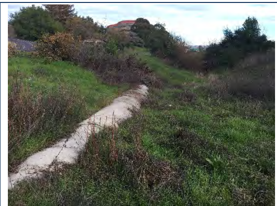
Partially exposed concrete storm drain pipe
