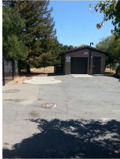
PHOTO 6 – ADJACENT PUMP HOUSE.
