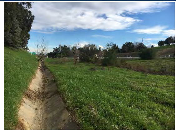
Concrete-lined drainage ditch on northeasterly portion of property
