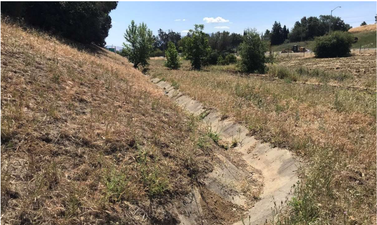
Photograph 8. Concrete ditch outside the eastern edge of study area, facing southeast.
